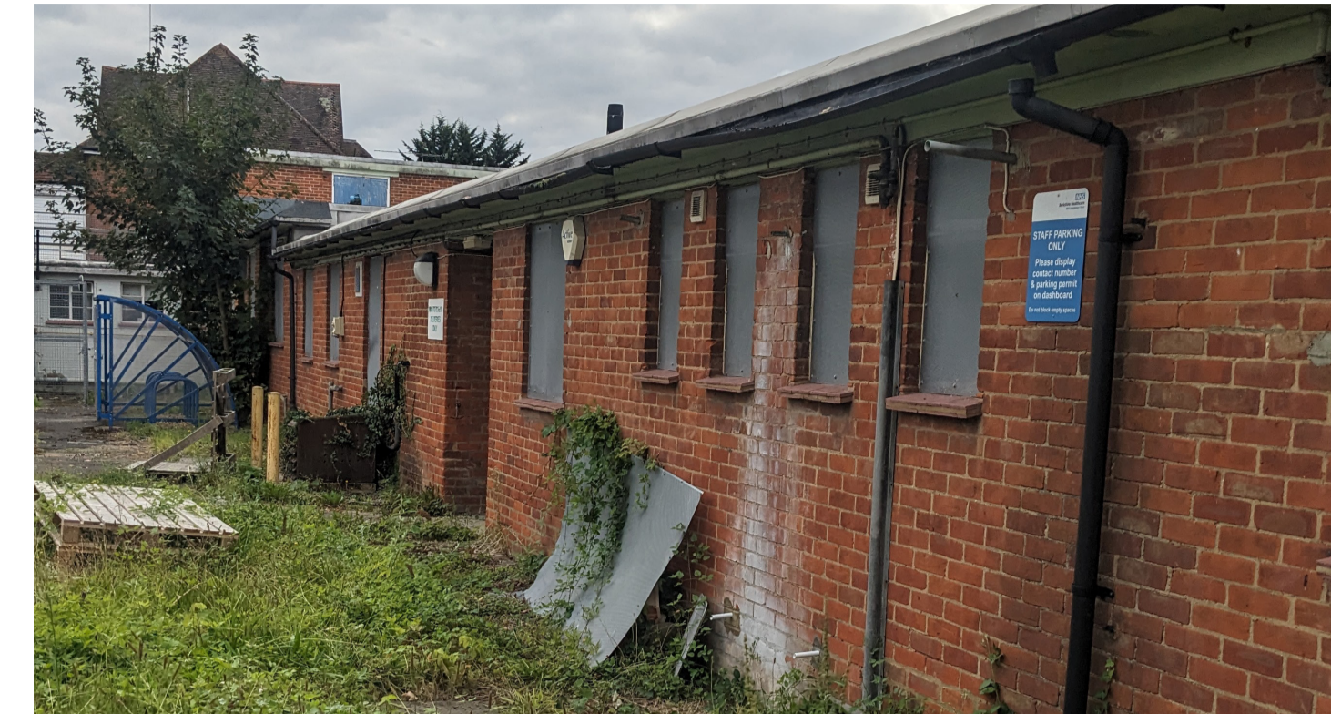
Another block which is to be demolished
