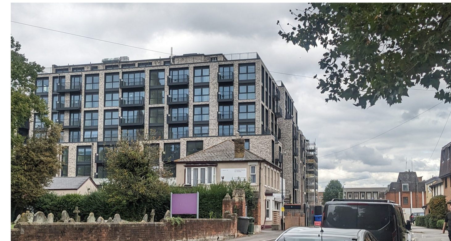
New block of flats on Church Street
