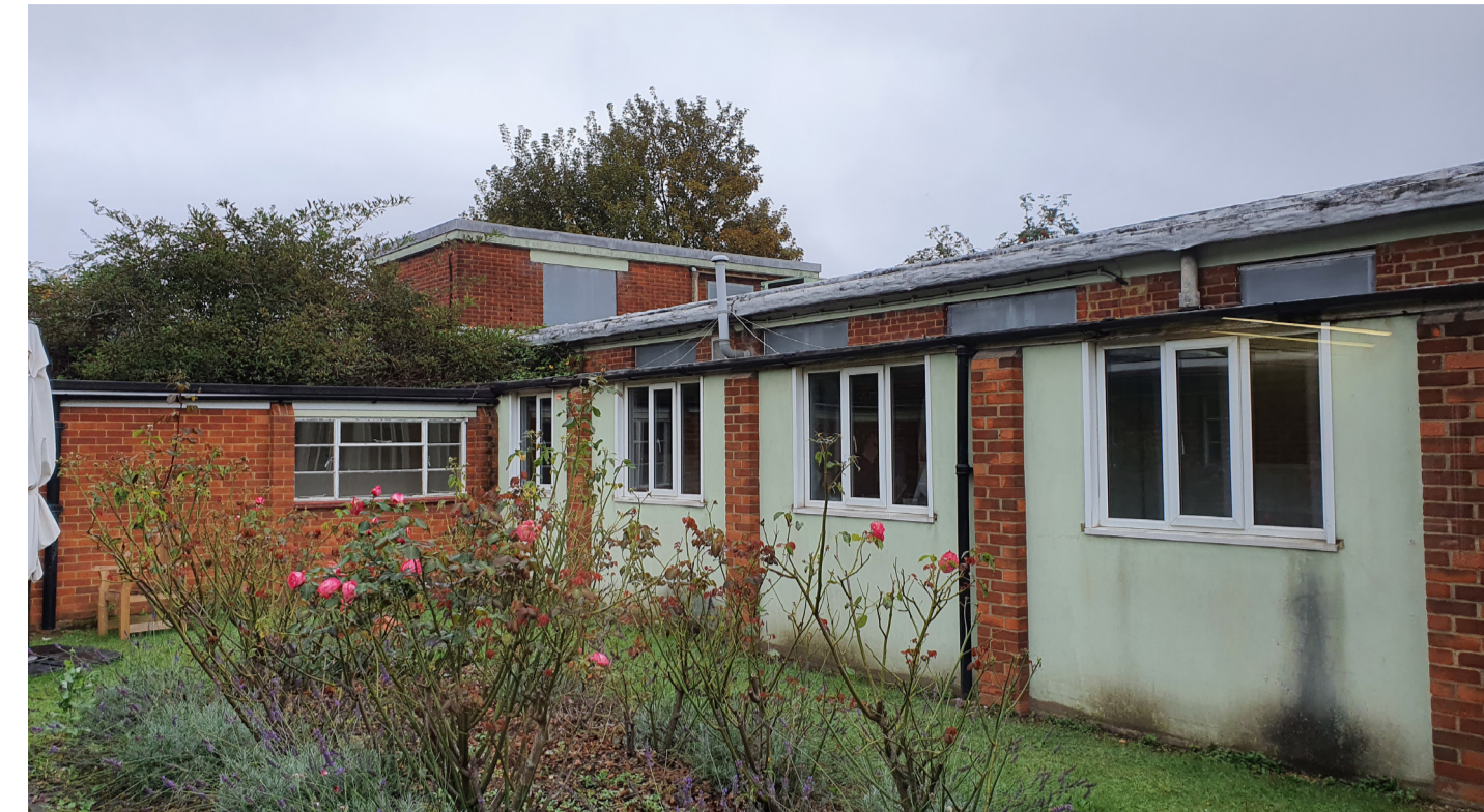
One of the vacant blocks to be demolished
