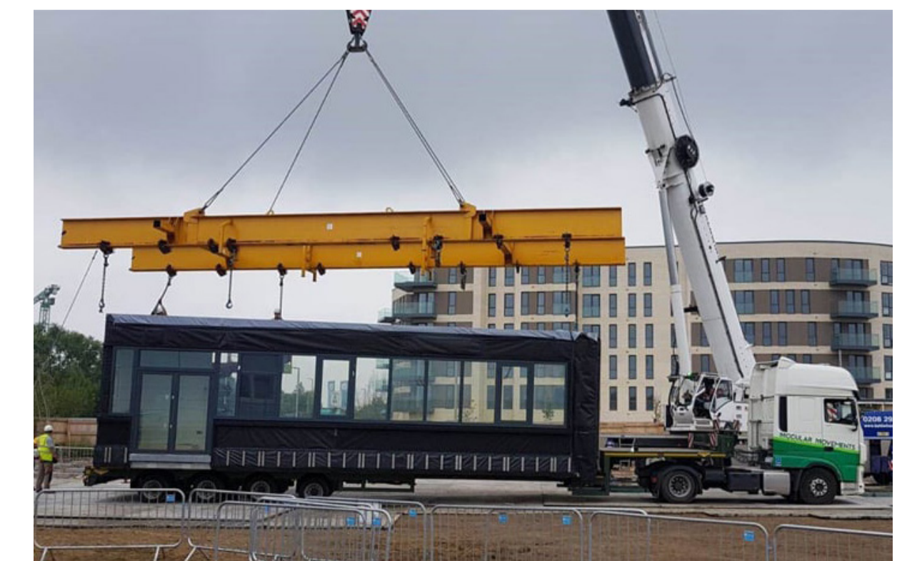
Examples of modular construction in the factory and on site
